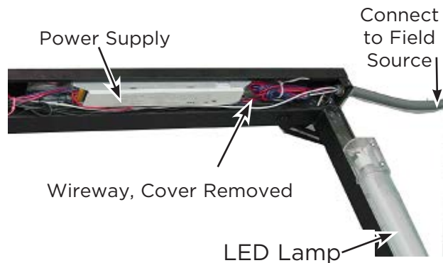
Connect Wireway Wiring to Power Source
