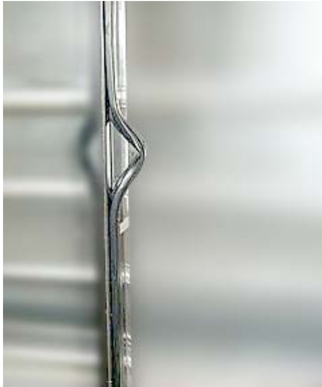
Improperly Installed or Damaged Gasket
