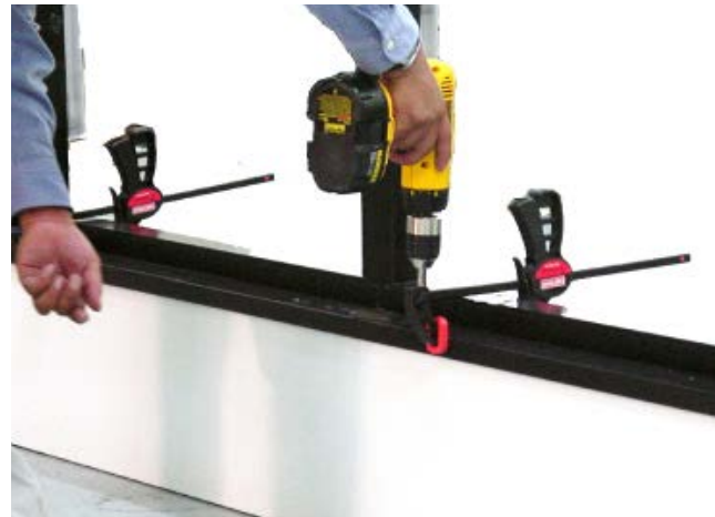
Fasten the Frame Bottom
