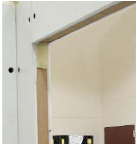
Standard Reinforced Opening frame.
