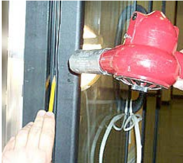
Pulling Gasket Into Place With a Pencil SERVICE AND MAINTENANCE Replacing Doors
