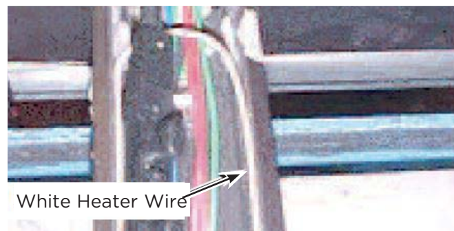
Remove and Replace Frame Heater
