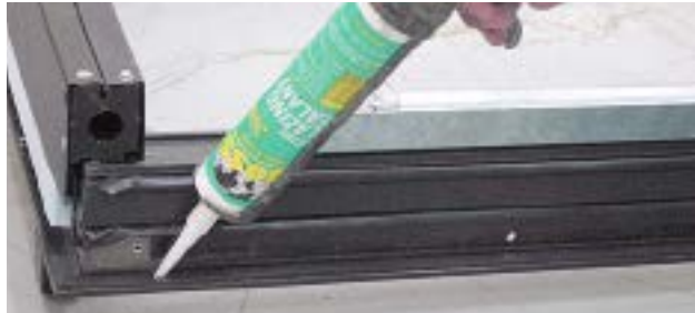
Apply Silicone Sealant
