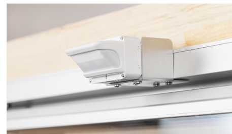
Ambient Sensors & LED Motion Sensor Installed
